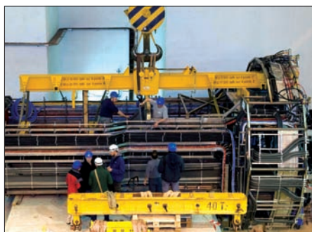
ALICE's “mini” space frame, which carries all the supply cables for services.
